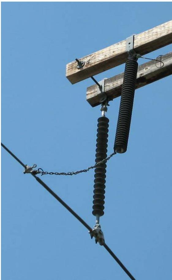
Figure 7 Lead Reinforcement with a chain
