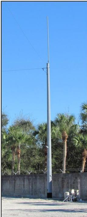
Figure 3 - Lightning Terminal in Substation
