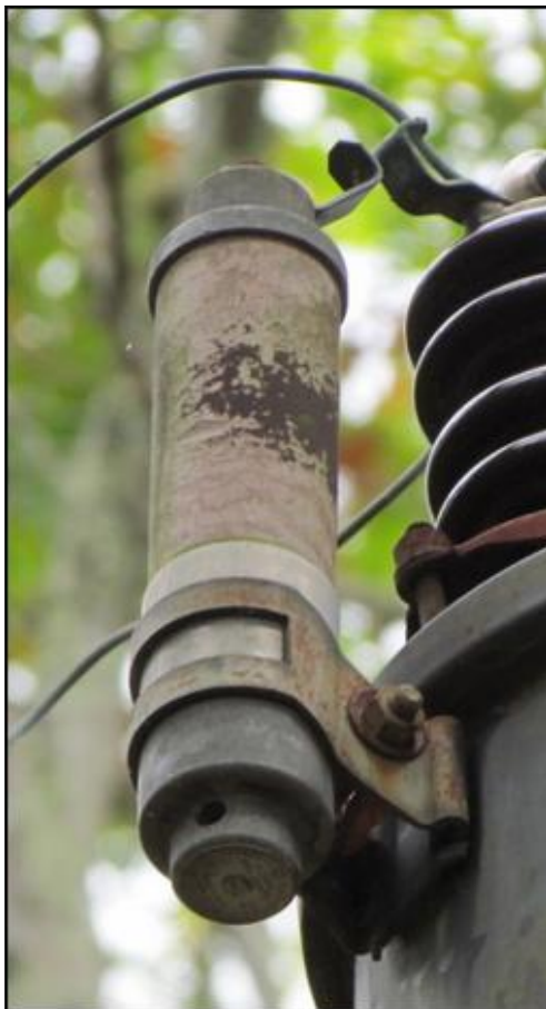
Figure 4 Another "Half Century Sentry". 1950 Hi-Stroke Rural Arrester by GE Still in service Oct 2011
