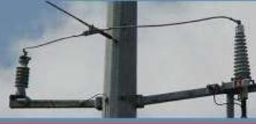
The title of this 1939 patent was Automatic Current-Interrupting Device. In 1939 the available fault currents on distribution systems was not more than a few thousand amps. This is the reason this device could interrupt fault current then and not today. Even today, the common models of ground lead disconnectors that use an explosive material to separate the ground lead can interrupt currents below a few thousand amps, but not system currents of 4000 amps or more.
